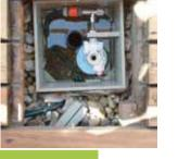
DHA-110-D Roof Outlet with height adjustable water level control
