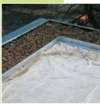
Where the roof does not rainwater to the drainage have a perimeter parapet wall, the RDT Edge Profile provides one possible solution to the problem of how to retain the garden elements, whilst still allowing the free flow of is achieved by means of
