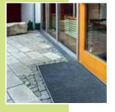
for clients to demand level access from their building to the adjoining terrace. This structure removes the danger creates detailing difficulties of any build up in this crucial with regard to ensuring there is area by feeding the rainwater no water ingress. One directly into the drainage possible solution is to use the system. It is essential that
